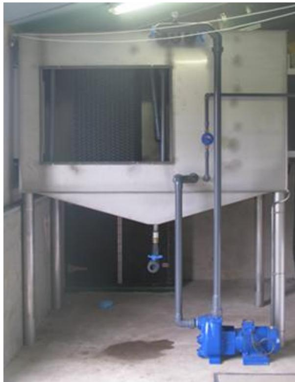
Development of a « one-third » bioscrubber and operating in breeding conditions with partial pit ventilation (33%)
